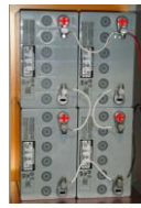
24V 102Ah Battery Configuration
