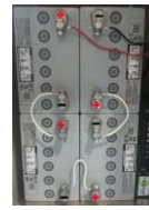
48V 51Ah Battery Configuration
