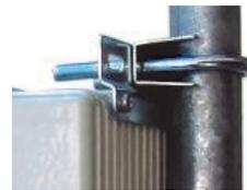
**STEP 1:** Install the unit to a suitable pole using included hardware. First install the brackets to the back of the enclosure using the screws provided. Next install the u-bolts and pole clamps. Note: the unit can be installed to a wall by setting aside the u-bolts and pole clamps and just screwing the mounting brackets to a wall.
